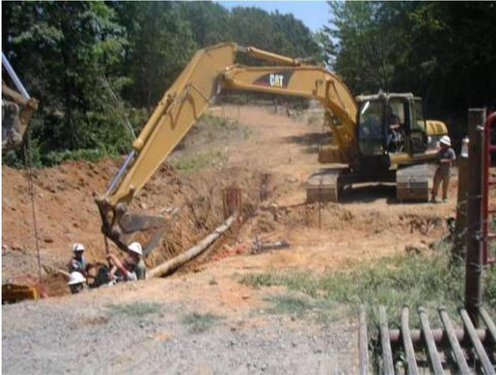
Figure 20 – Worker connecting pipeline sections. Pipeline corridor can be seen in the background.
