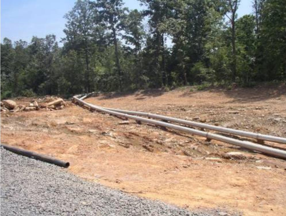
Figure 10 – Water pipeline conveying water for a frac job.
