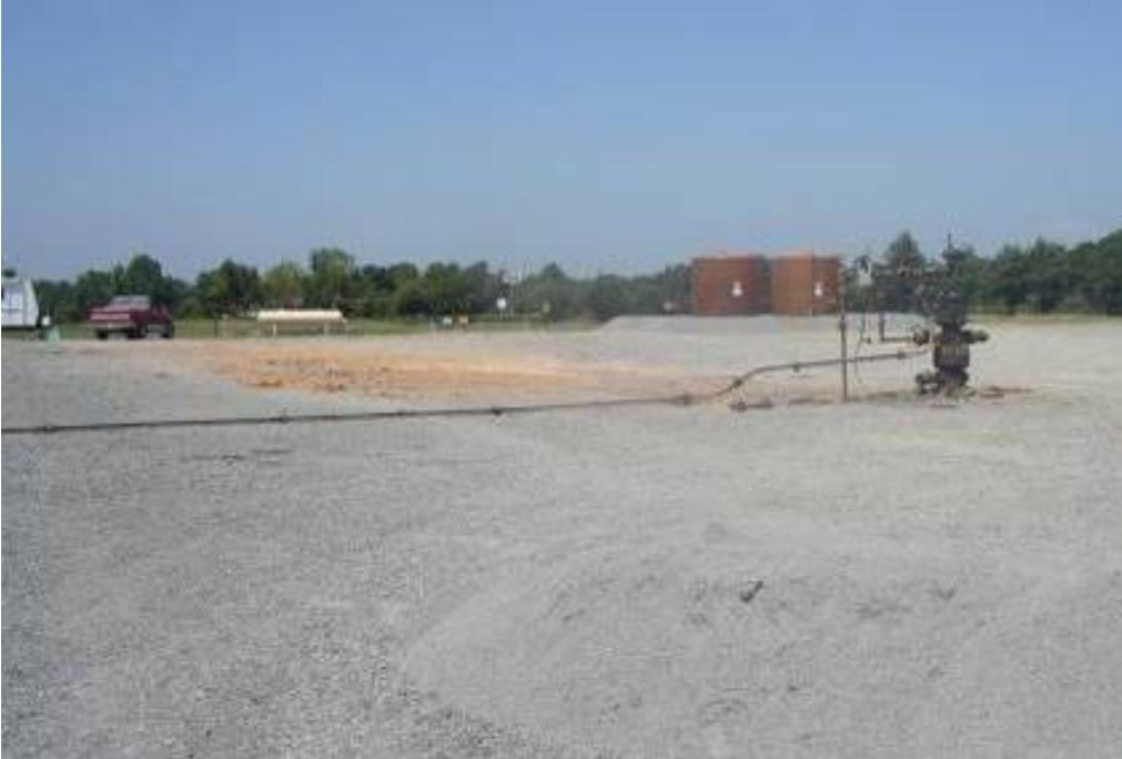
Figure 2 – Newly constructed well showing gravel pad.
