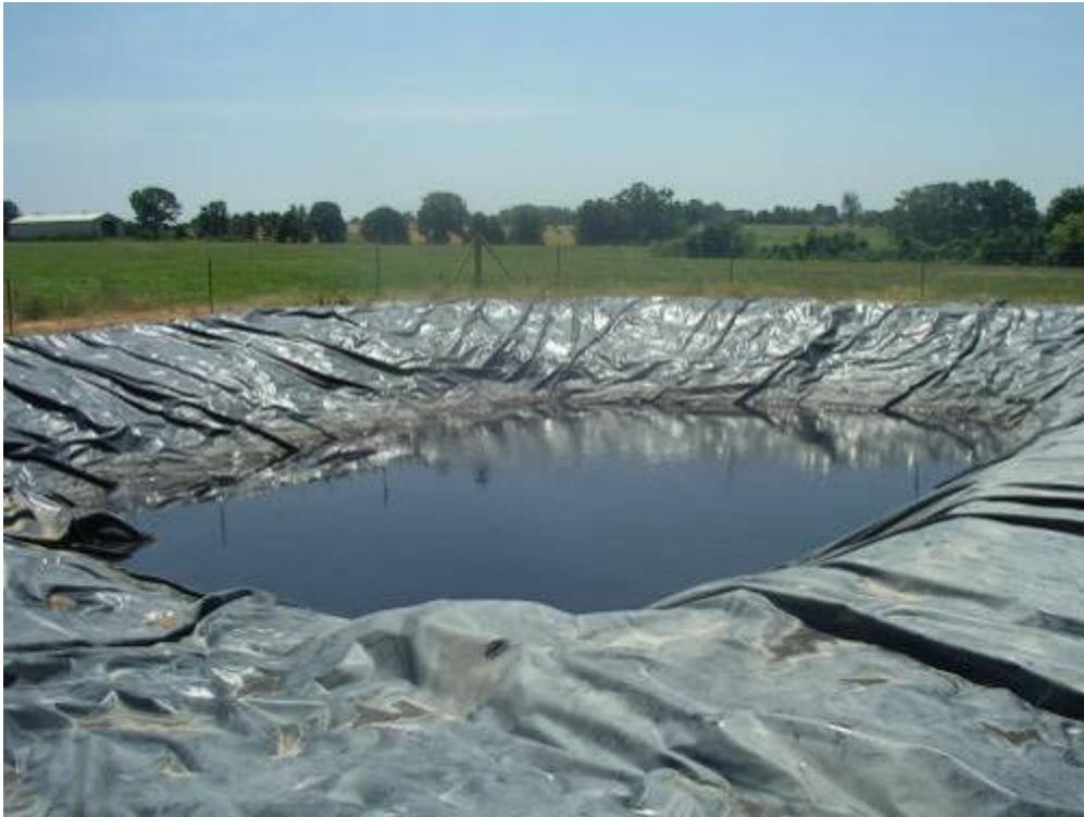
Figure 5 – Rig ditch pit.
