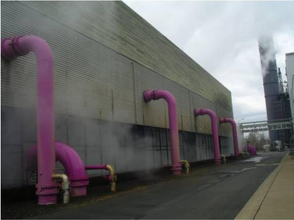
**Figure 7 – Reclaimed Water Pipe and Recirculating Pumps (Source: Veil 2007)**
