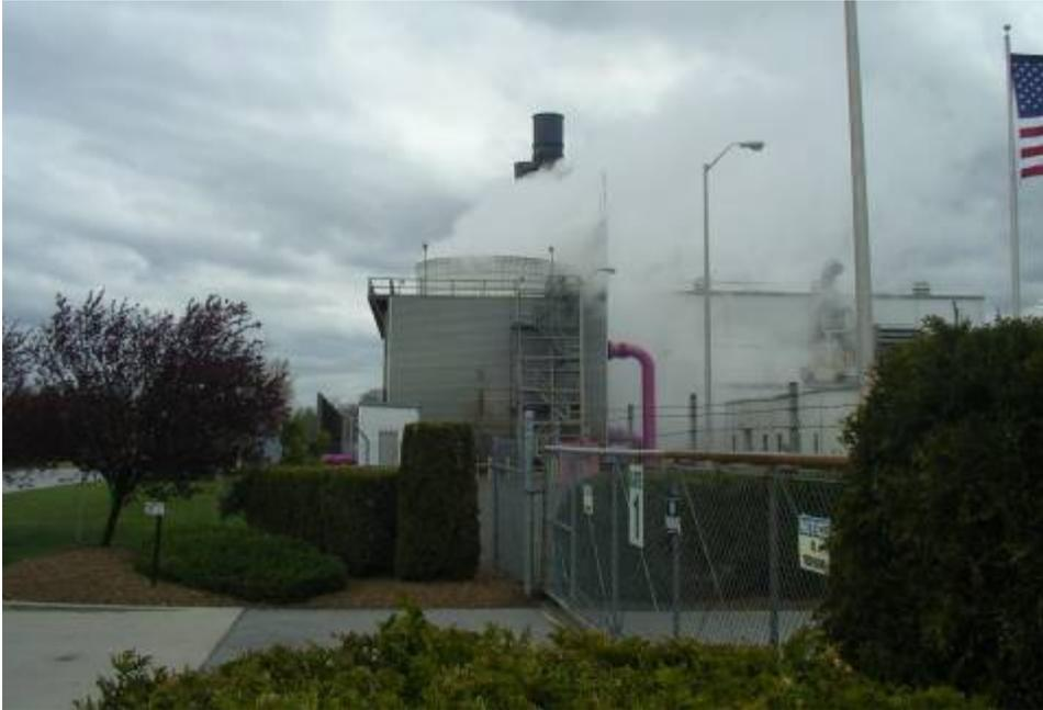
**Figure 9 – Reclaimed Water Falling through Cooling Tower and Forming a Mist (Source: Veil 2007)**
