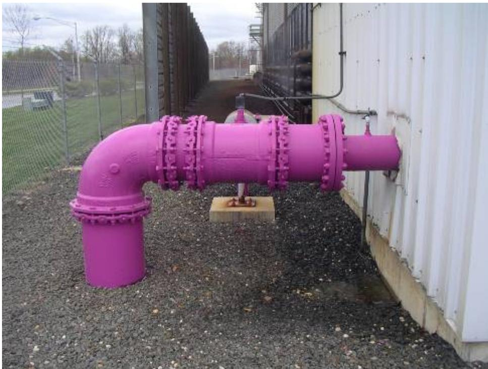
**Figure 6 – Reclaimed Water Lines and Cooling Tower (Source: Veil 2007)**
